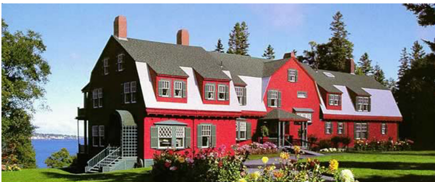
Main Lodge House, Campobello
